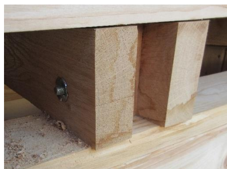
Vissage support/traverse
